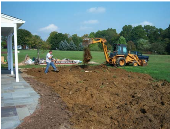
A backhoe used to break compaction.
