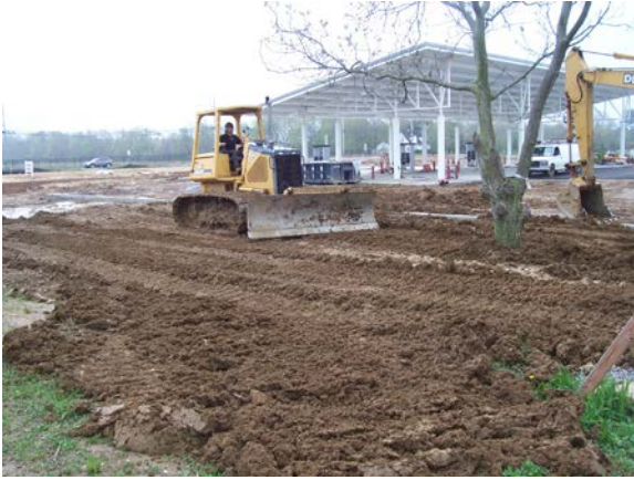
Soil compaction caused by construction equipment.
