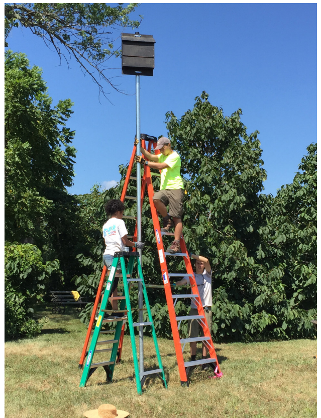
Figure 3. Installation of a pole-mounted bat house. (Photo Credit: Brooke Maslo)
