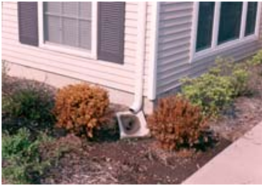
Figure 3. Yew plants affected by excessive moisture. (Photo courtesy R. Buckley)
