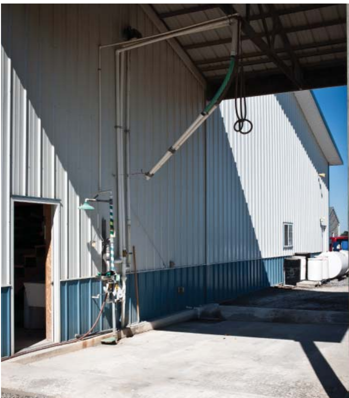
Left: A pesticide fill area. The impervious pad has a curb to contain any spills.
