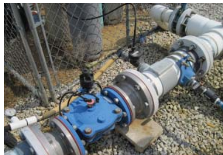
Above, top: Chlorine gas treatment system, with cage for protection
